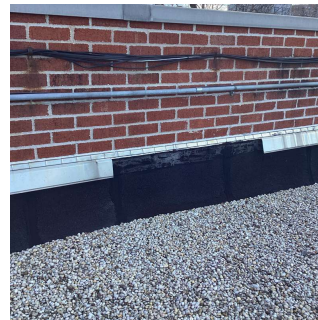
Roof 1 - Facade A
