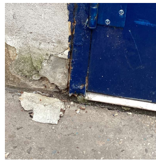
Facade K - Near Exit 8 No violations recorded.
