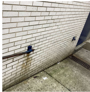
Facade K - Near Exit 8
