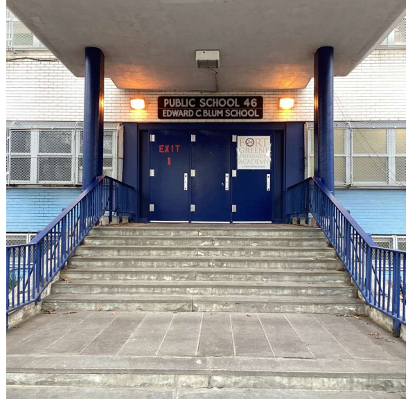
Facade A - Clermont Avenue
