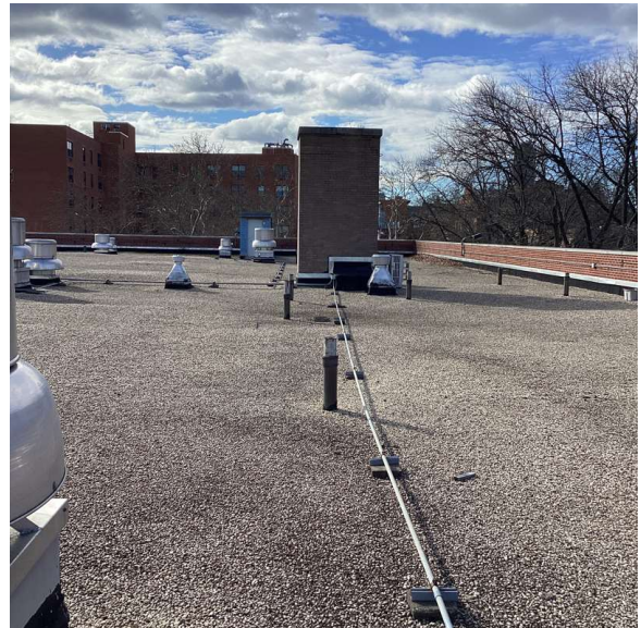
Roof 1 - South View
