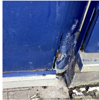
Facade H - Exit 15
