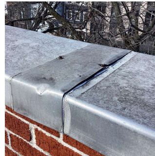
Roof 1 - Facade C No violations recorded.
