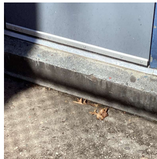
Facade B - Exit 3
