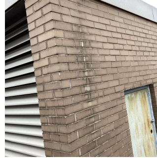
Shaft Vent Brick
