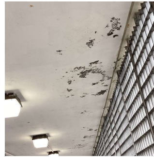
2nd, 3rd Floor Exterior Walkways
