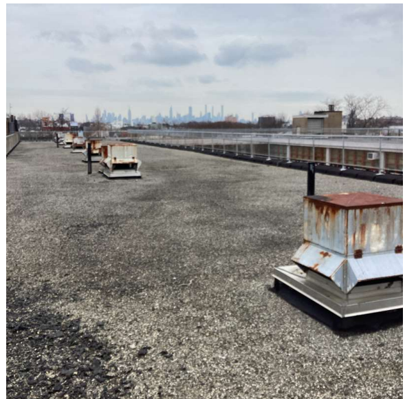
Roof 1 - North View
