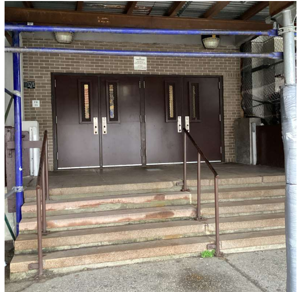
Facade A - Emmons Avenue
