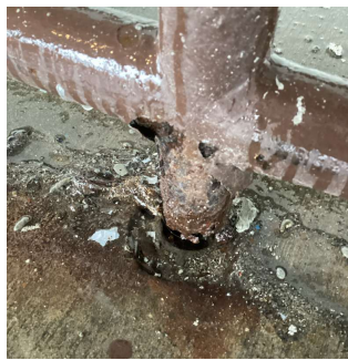
Facade A No violations recorded.
