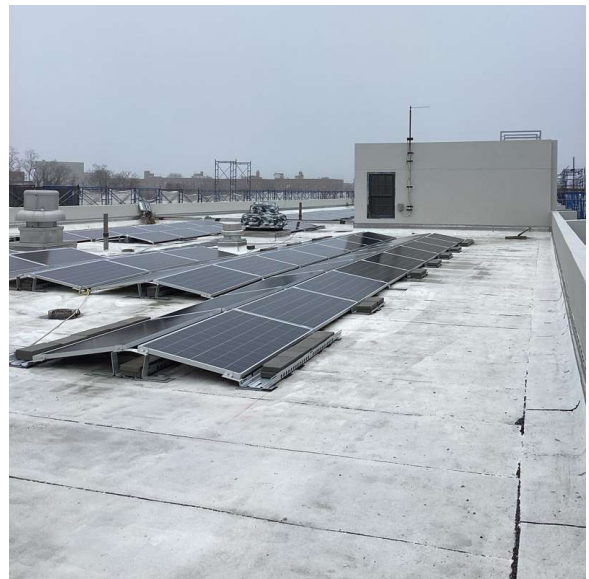
Roof 1 - Northwest View
