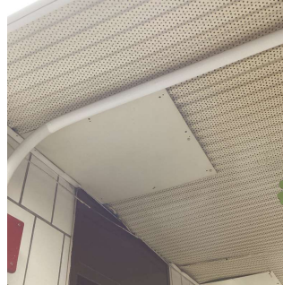
Corridor near Room 408
