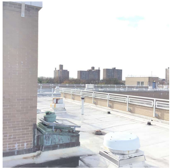
Roof 1 - South View
