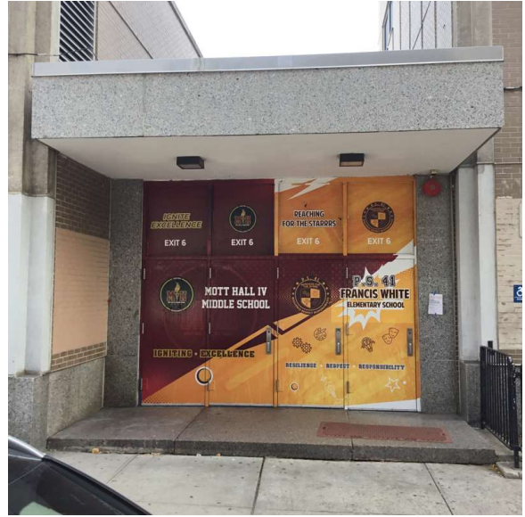
Facade A - Thatford Avenue
