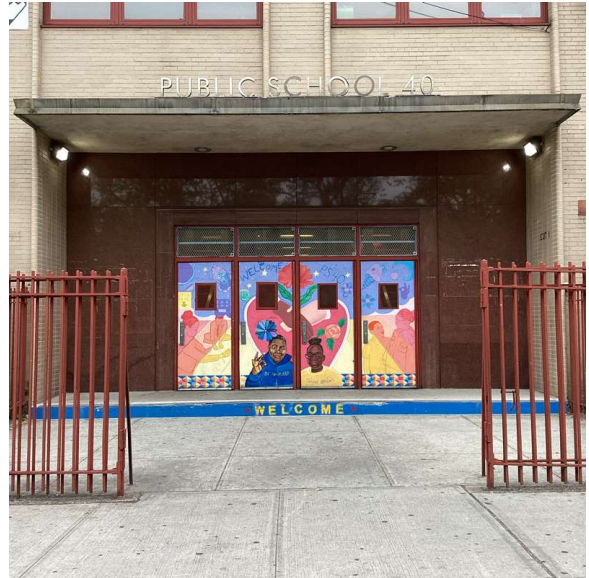
Facade A - Ralph Avenue
