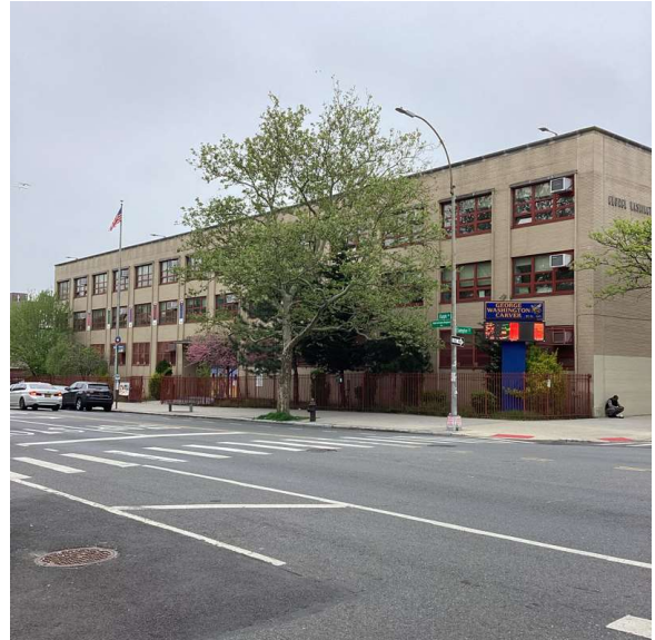
Corner of Ralph Avenue and Sumpter Street - Northeast View
