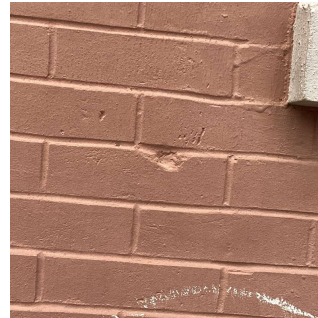
Facade D - Near AW2
