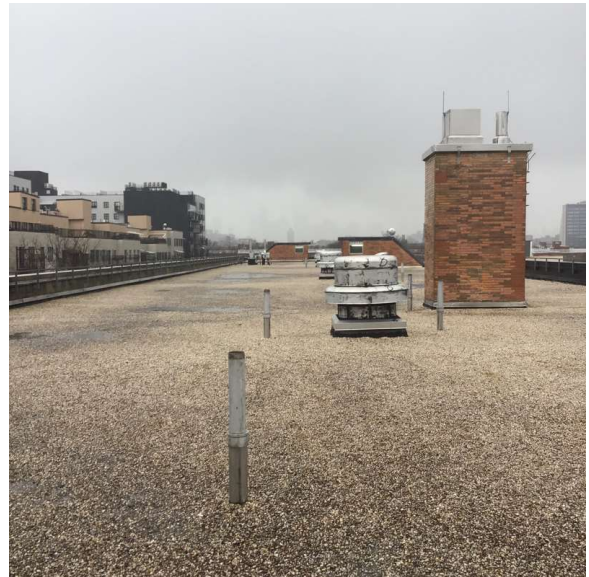
Roof 1 - West View
