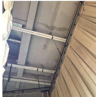
Roof 3 - Auditorium Stage (shown), Gymnasium, Roof 1 - Room 431, Stairs A/4, B/4
