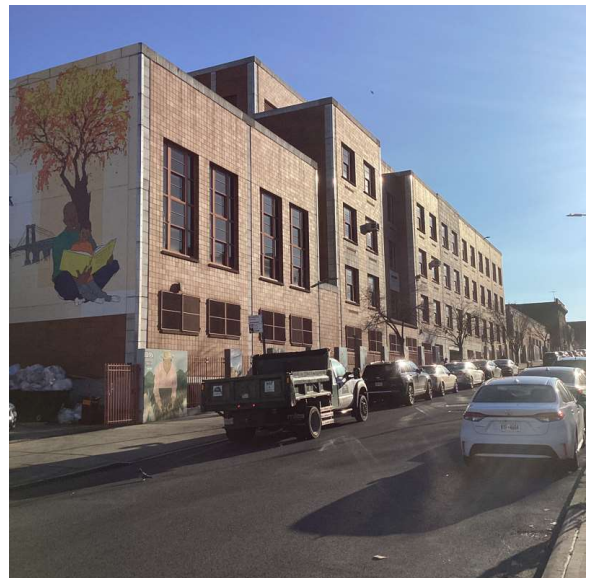
Corner of 38th Street and 4th Avenue - East View
