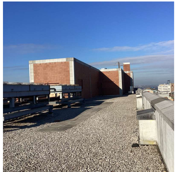
Roof 1 - West View
