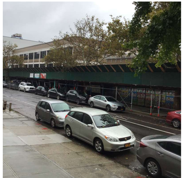
Corner of Willoughby Avenue and Tompkins Avenue - West View
