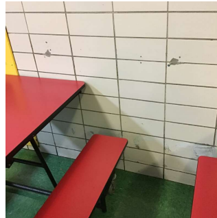
Rear Near Windows
