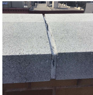
Facade A - PH3 No violations recorded.
