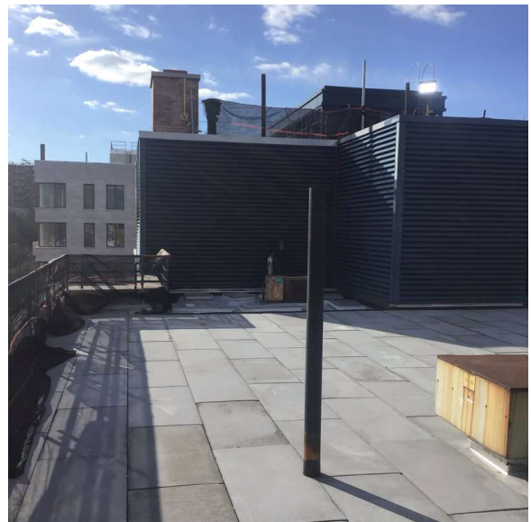
Roof 1 - South View
