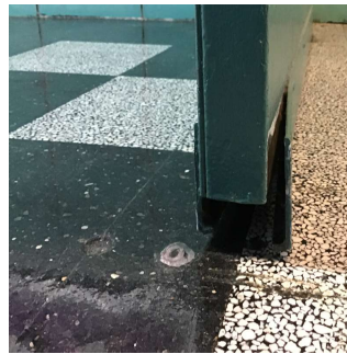
Corridor near Cafeteria
