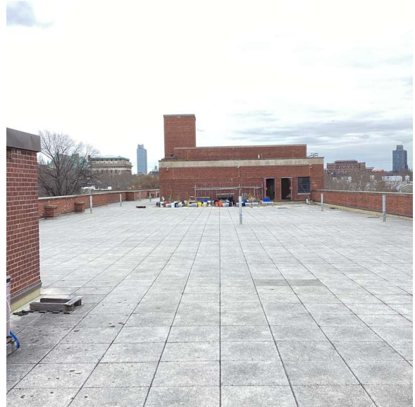
Roof 1 - South View
