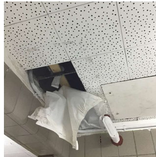
Corridor near 1st Floor Boys Toilet
