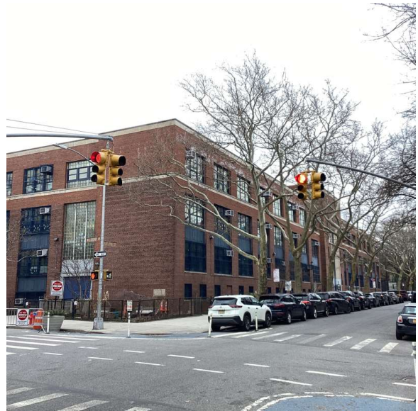
Corner of Adelphi Street and Willoughby Avenue - South View
