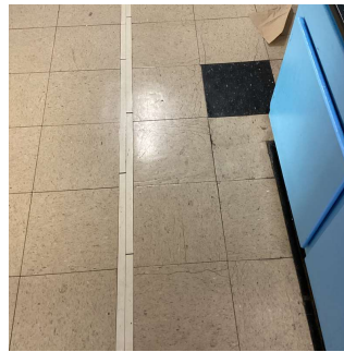
Corridor near Room 403
