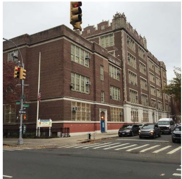
Corner of Wilson Street and Bedford Avenue - North View
