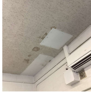
Near Main Entrance
