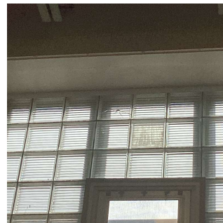
Facade D - Gymnasium
