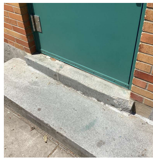
Facade E - Exit 4 No violations recorded.
