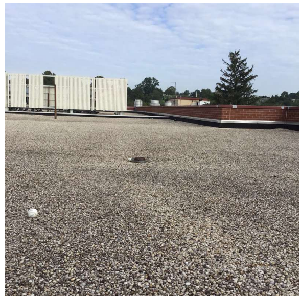
Roof 1 - North View
