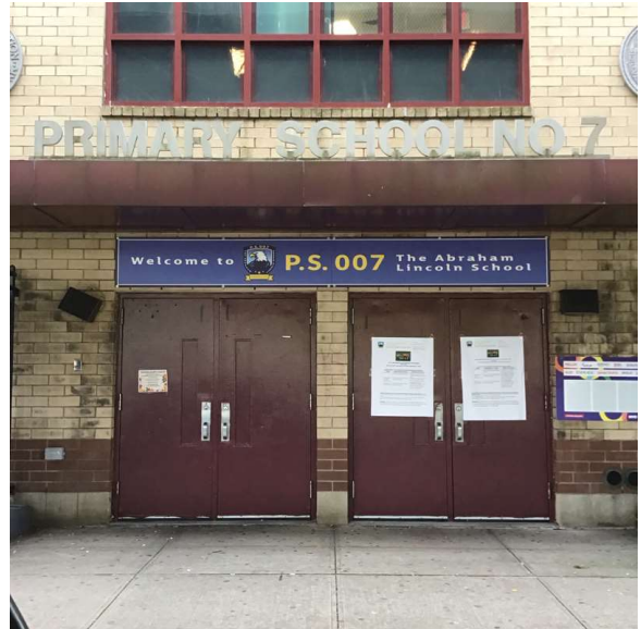
Facade A - Jamaica Avenue
