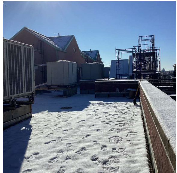
Roof 1 - South View
