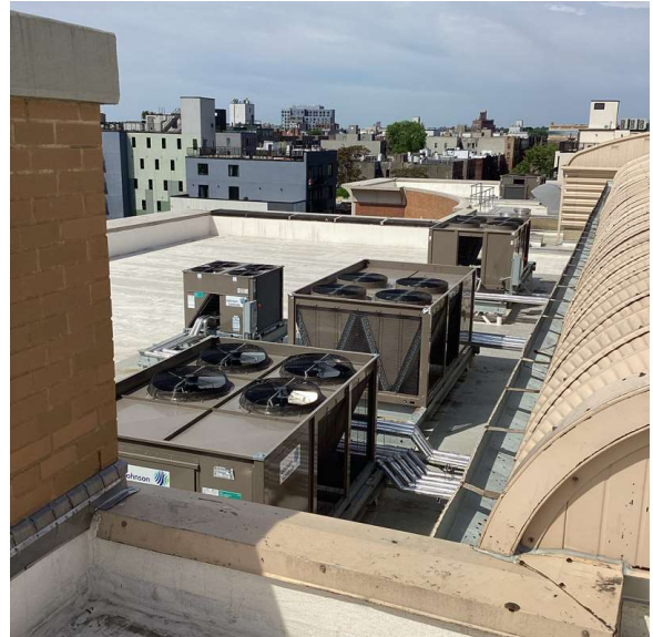
Roof 1 - Southwest View
