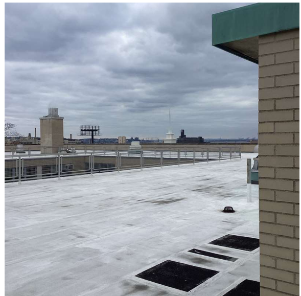
Roof 1 - West View
