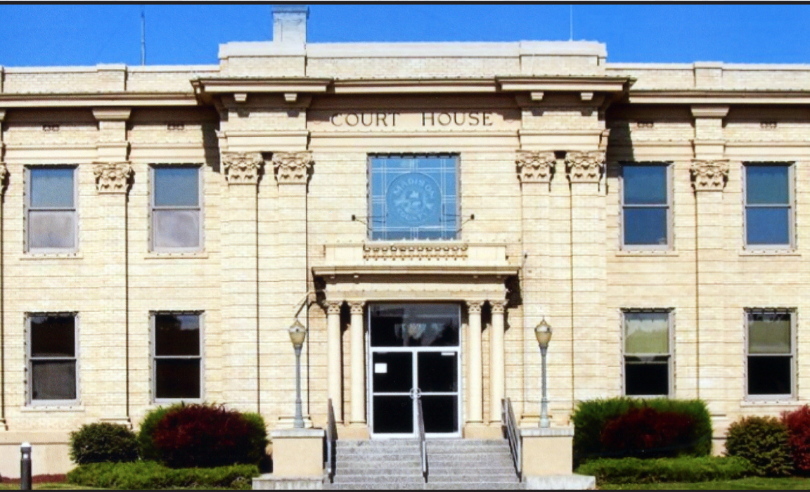
Madison County Courthouse
