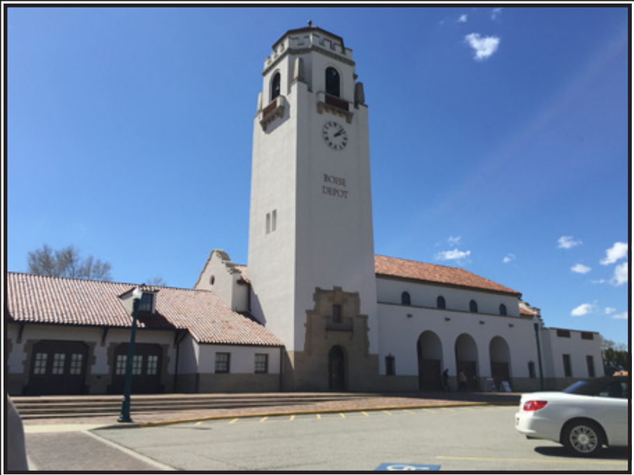
Union Pacific Mainline Depot
