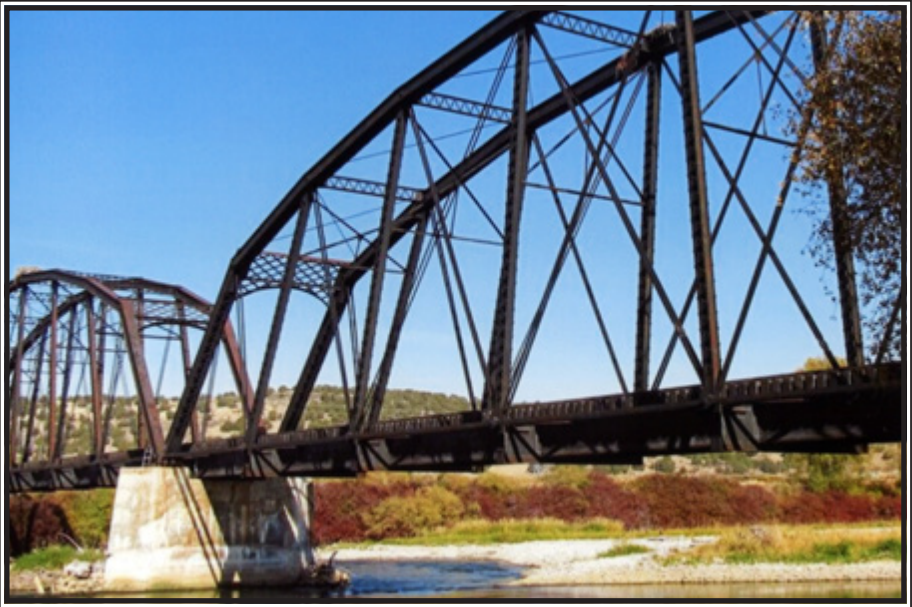
Ririe Pegram Truss Railroad Bridge
