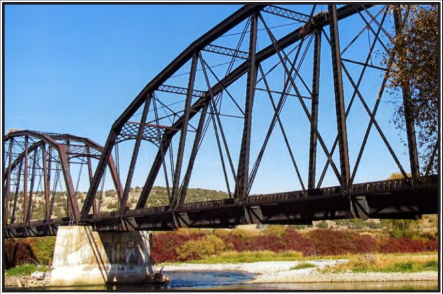
Ririe Pegram Truss Railroad Bridge
