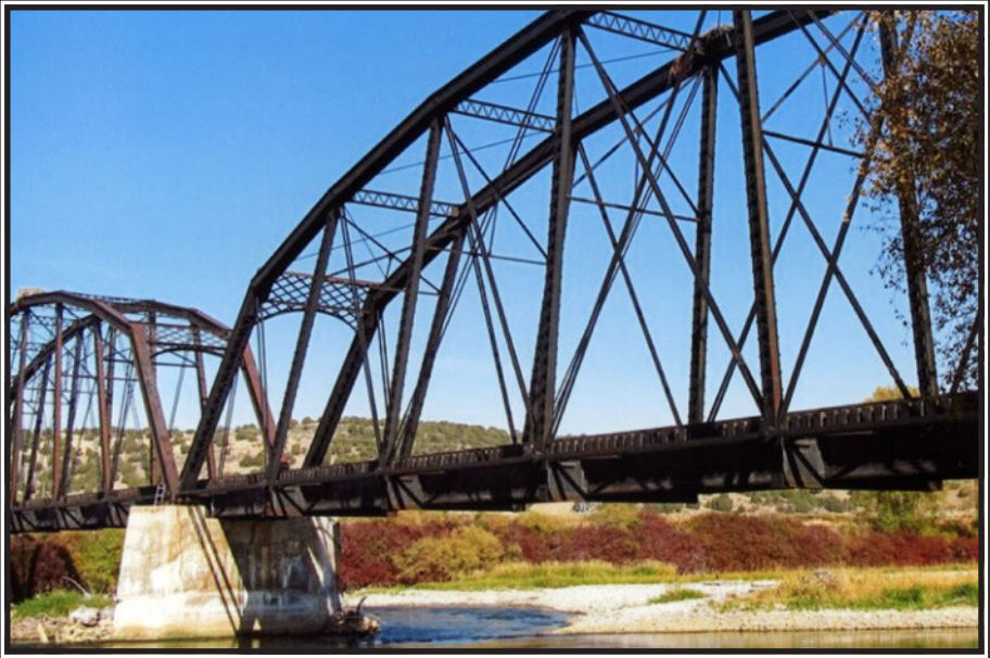
Ririe Pegram Truss Railroad Bridge
