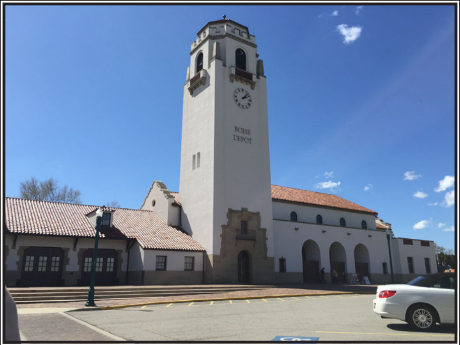
Union Pacific Mainline Depot
