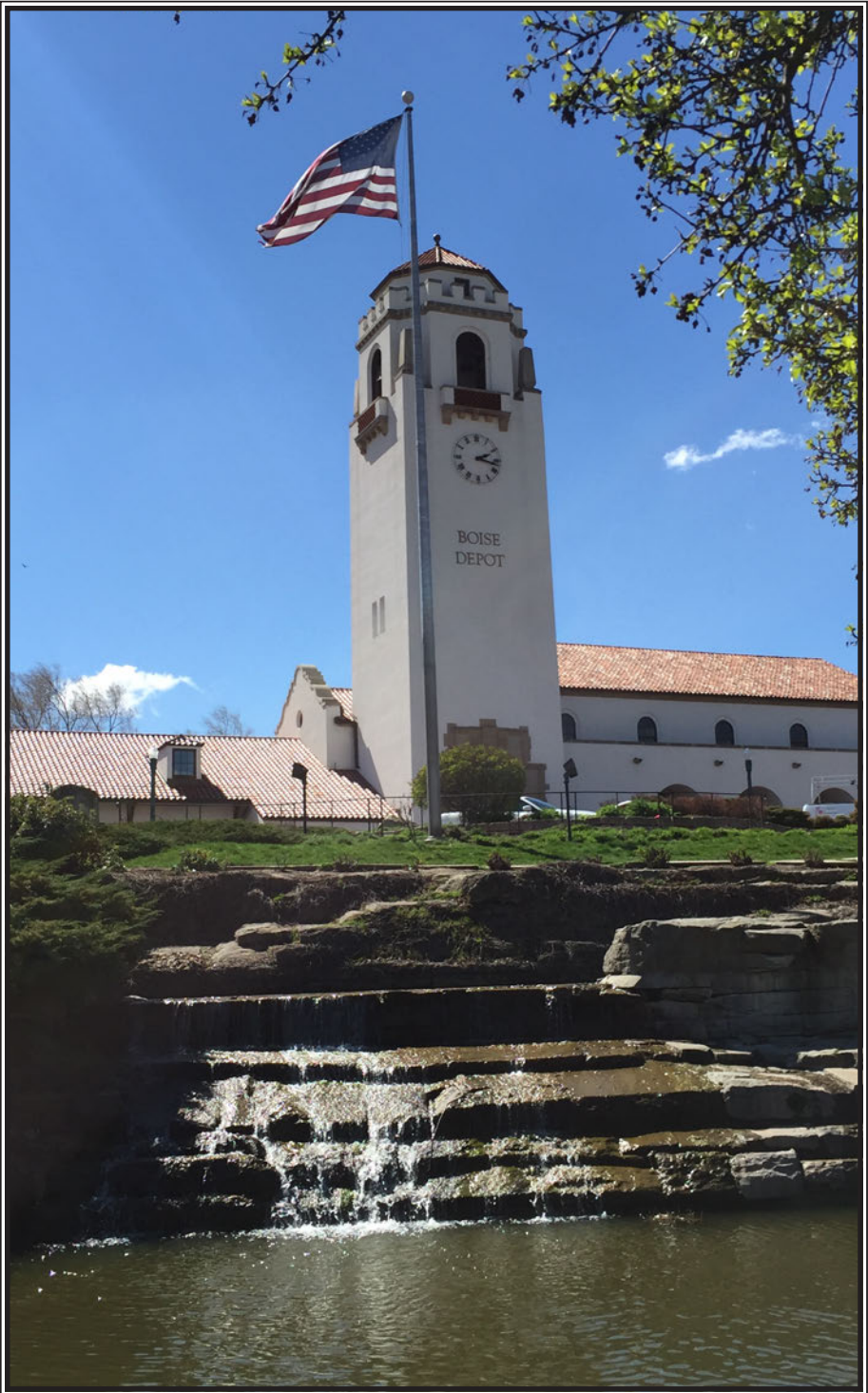
Union Pacific Mainline Depot
