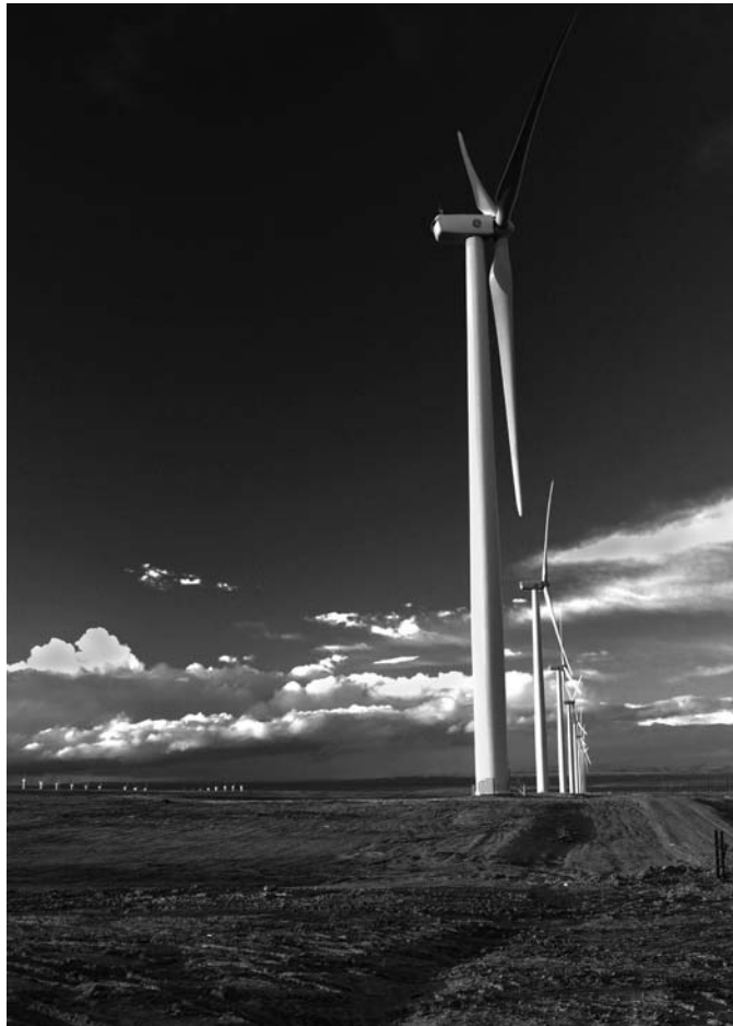
Wind Power Generation
