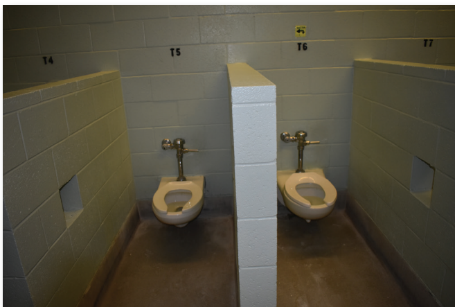
Figure 4. Toilets, Golden State.
