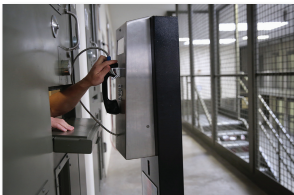
Figure 16. Use of Telephones at Men’s Restricted Housing Unit, Adelanto.
