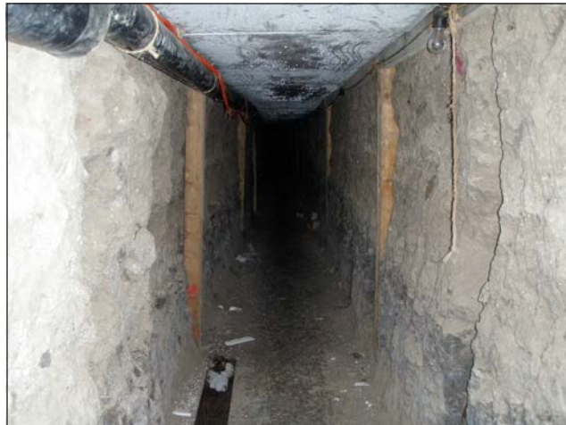
This tunnel, discovered in 2011, was used for trafficking drugs across the border and resembles other tunnels that can be used for the trafficking of persons. It ran more than 600 yards and was equipped with electric rail cars, lighting, reinforced walls, and wooden floors. The tunnel also had hydraulic doors and an elevator.
