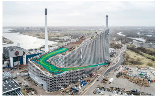
BIG's Amager Bakke/Copenhill, a ski slope and climbing wall on a waste-to-energy plant in Copenhagen
