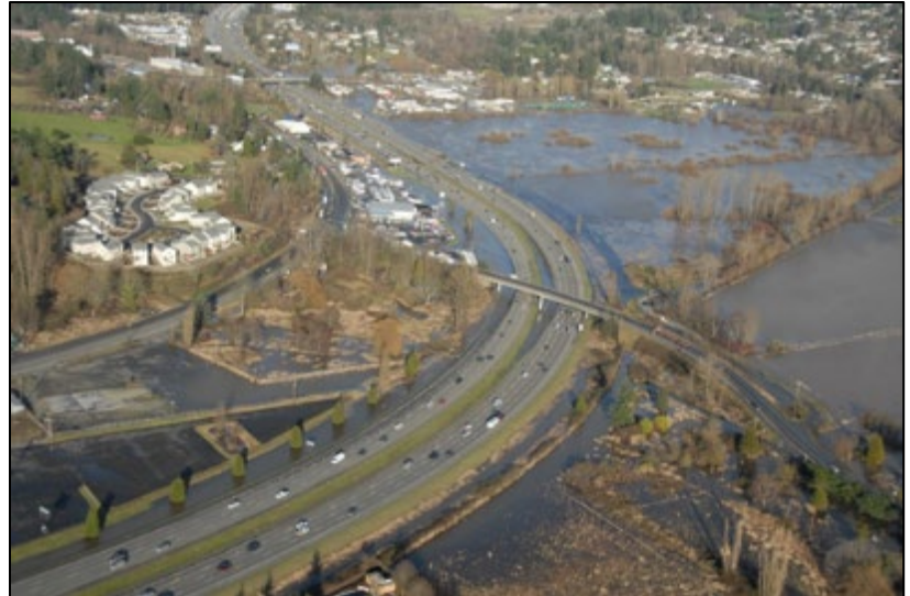
Figure 22: Flooding of Hylebos Creek around I-5 near the 70 Street over crossing (Fife Curve) in 2009 (Source: WSDOT).
