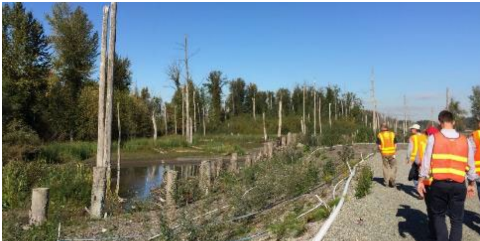
Figure 24: Delegation members walk along the new White River levee, which King County shifted out further from the river to allow for flood storage and habitat restoration. (Source: WSDOT).
