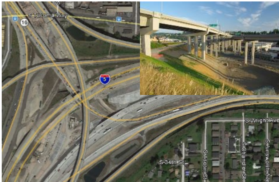
Figure 18: Conventional stormwater detention ponds under the I-5/SR 16 interchange. Due to the topography, shown on the inset, the detention pond is not located in an area with shallow groundwater and the topography provides the hydraulic head to evacuate the pond prior to a subsequent precipitation event. (Source: WSDOT).
