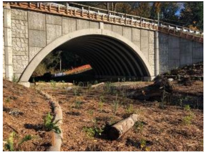
Figure 5: Fish passage project at SR203 Loutis Creek (Source: WSDOT)
