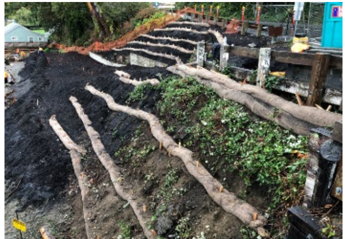
Figure 6: Tahlequah slope stabilization project (Source: WSDOT)
