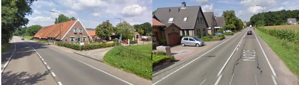
Figure 77 N225 in 2010 during the road works
