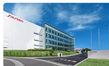
Osaka Ibaraki factory and neighboring West Japan Distribution Center
