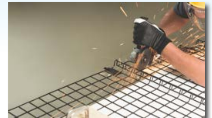
Safety panels are easily cut in the field for custom-size panels
