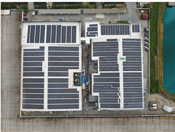
A 1452 kilowatt project, consisting of 2,664 solar panels was installed atop the roofs of 2 facilities in Bangkok, Thailand. The project produced 1,918,709 kilowatt hours of electricity in its first year online (2022).
