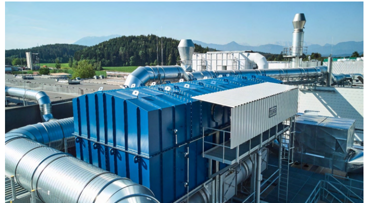
CCL Label invested in a new regenerative thermal oxidizer (RTO) at our Völkermarkt site in Austria that supports us in realizing the lowest emissions possible in label and sleeve production. The RTO functions as a centralized system for the entire production process and provides a total air volume up to 60.000 m3/h.
