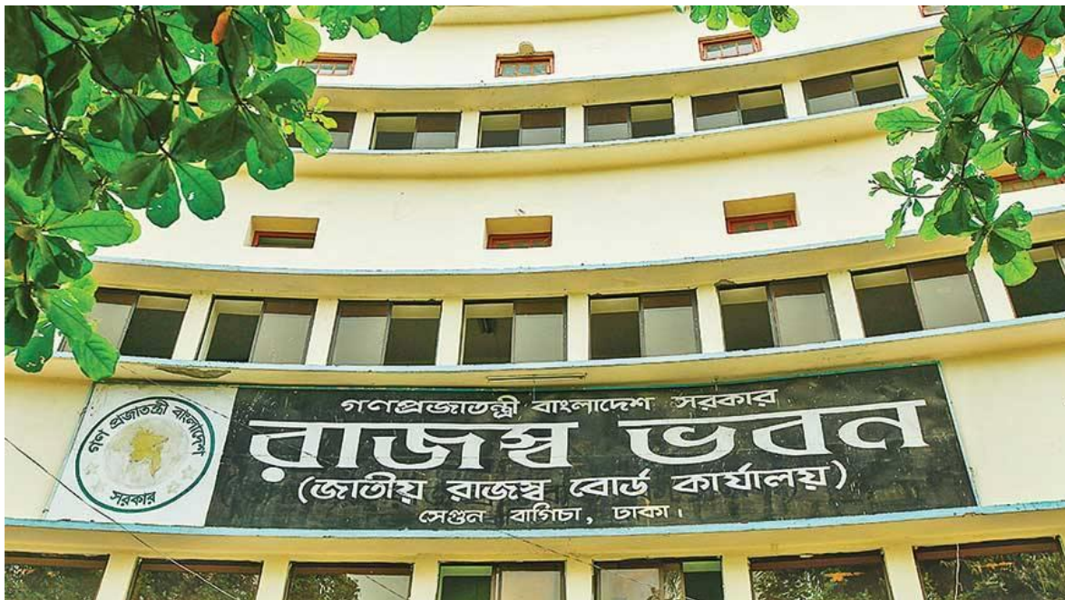
Figure 16: National Board Revenue Headquarter in Dhaka
