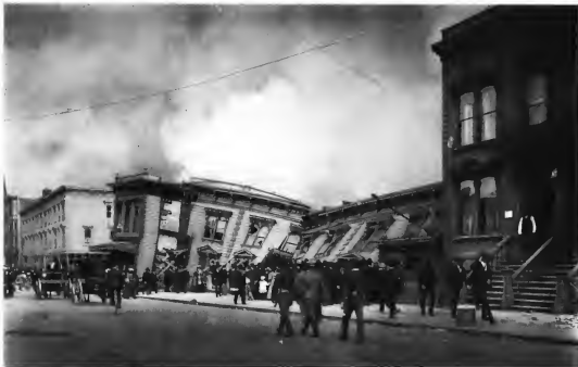
Golden Gate Avenue, near Hyde Street, San Francisco. An example of buildings that had been built on infirm (swampy) ground. When the 1906 earthquake hit, swampy ground turned into liquid—a suspension of dirt and sand in water.
