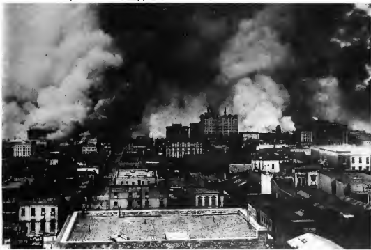
An example of a photo retouched to hide earthquake damage. Buildings with collapsed walls have been painted over to appear intact.
