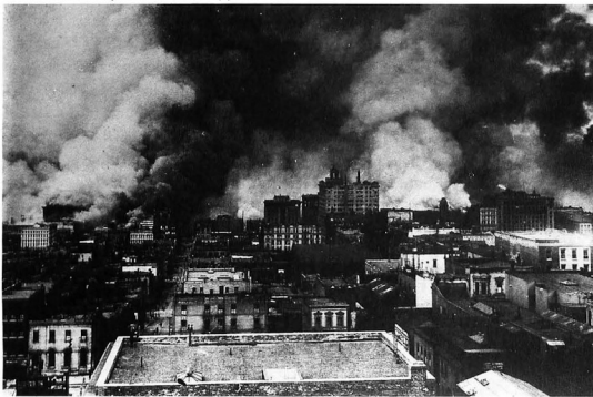
An example of a photo retouched to hide earthquake damage. Buildings with collapsed walls have been painted over to appear intact.
