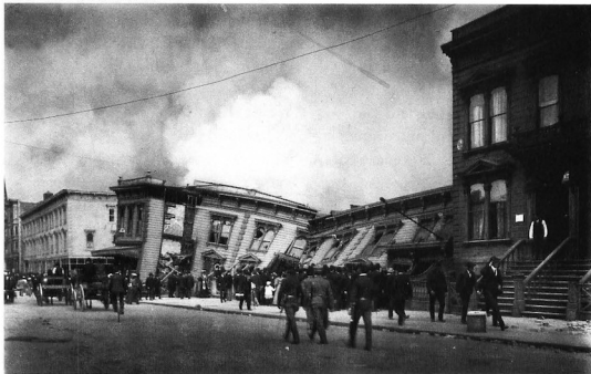
Golden Gate Avenue, near Hyde Street, San Francisco. An example of buildings that had been built on infirm (swampy) ground. When the 1906 earthquake hit, swampy ground turned into liquid—a suspension of dirt and sand in water.
