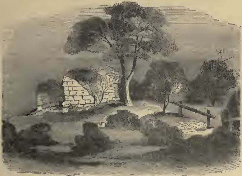
Clonsast Old Church, King's County.
