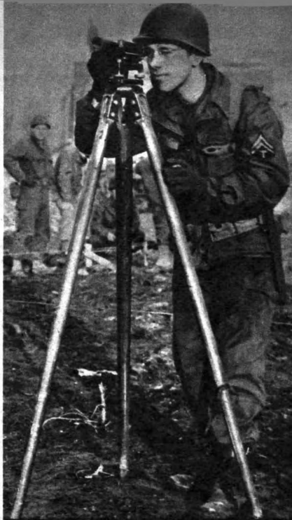
Cpl. Louis Rossano of Brooklyn, N. Y., surveys a cleared site in the Lambeth district of London before a prefabricated house is set up.
