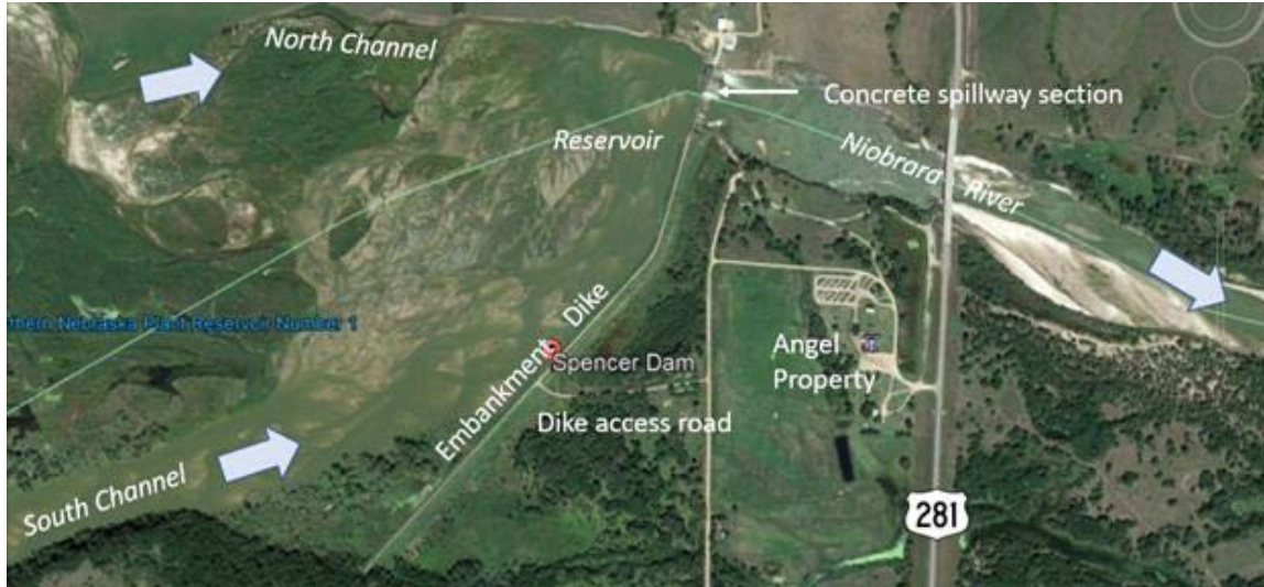
Figure 2. Aerial view of Spencer Dam and Vicinity (ASDSO, 2020).
